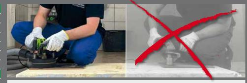
Due to dust exhaust best **protection of the user against dangerous mineral dusts,** compared to conventional methods with angle grinders
